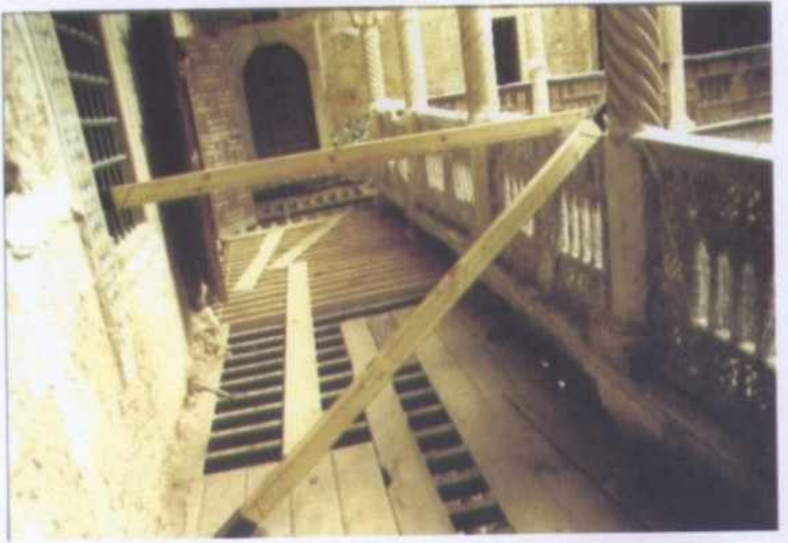
FIGURE 437 : DISPOSITION DES SOLIVES.
