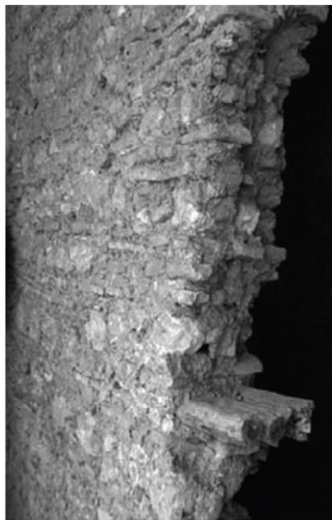
Figure 47 renforcement des murs (source: A.Foufa)
