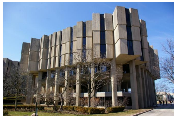
Figure 46. Northwestern University Library, Stack Tower, extérieur. Photo © 2014 Shawn Hazen.
