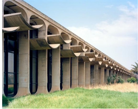
Figure 69. Bloc des Salles de Classe IV, Houari Boumediene University of Science and Technology, Bab Ezzouar, Algeria, 2013. Photo © 2018 jasonoddy.com
