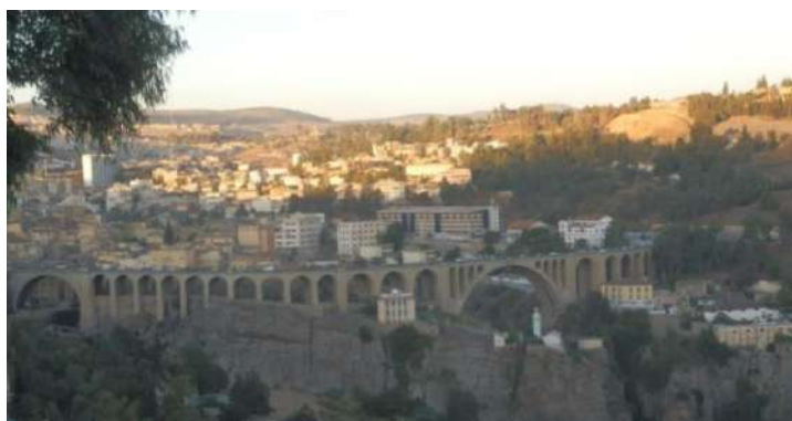
Fig. 65 Pont de Sidi Rached.
