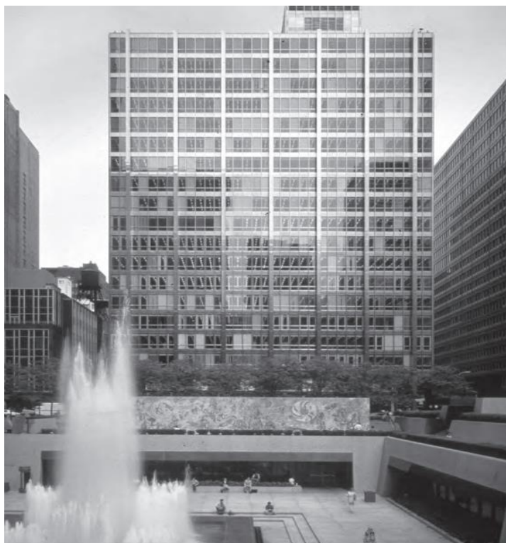
Figure 16: Inland steel Building, Chicago.
