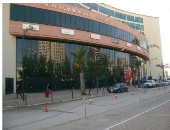
Figure -37- : Centre commercial - Bab-Ezzouar
