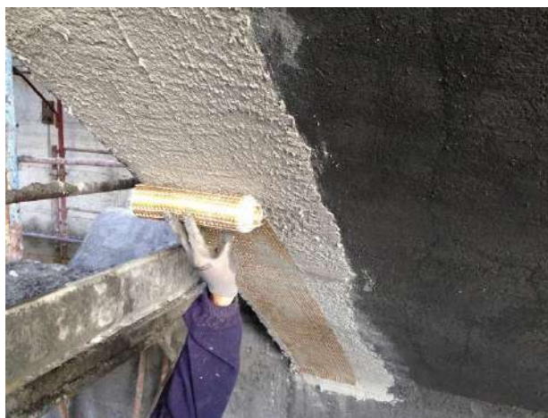
Fig 6.2.3 Application localisée du système FRCM (Source : https://www.edilportale.com/news/2017/06/aziende/i-sistemi-pbo-frcm-si-confermano-una-soluzione-efficace-per-i-rinforzi-strutturali_58506_5.html )
