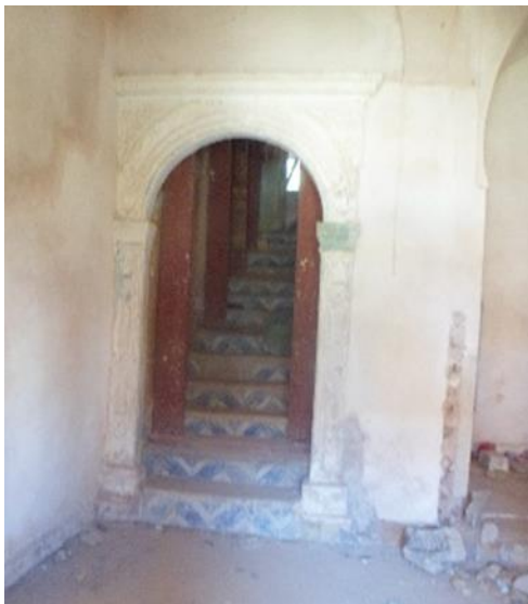
Figure 39: Escalier principal de la villa A (I.S.003)
