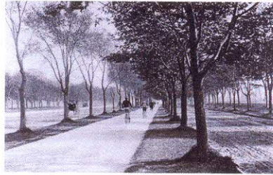
Figure1: Parkway 1894 The New Bicycle Path Ocean Parkway source: http://www.nycgovparks.org/about/history/olmsted-parks
