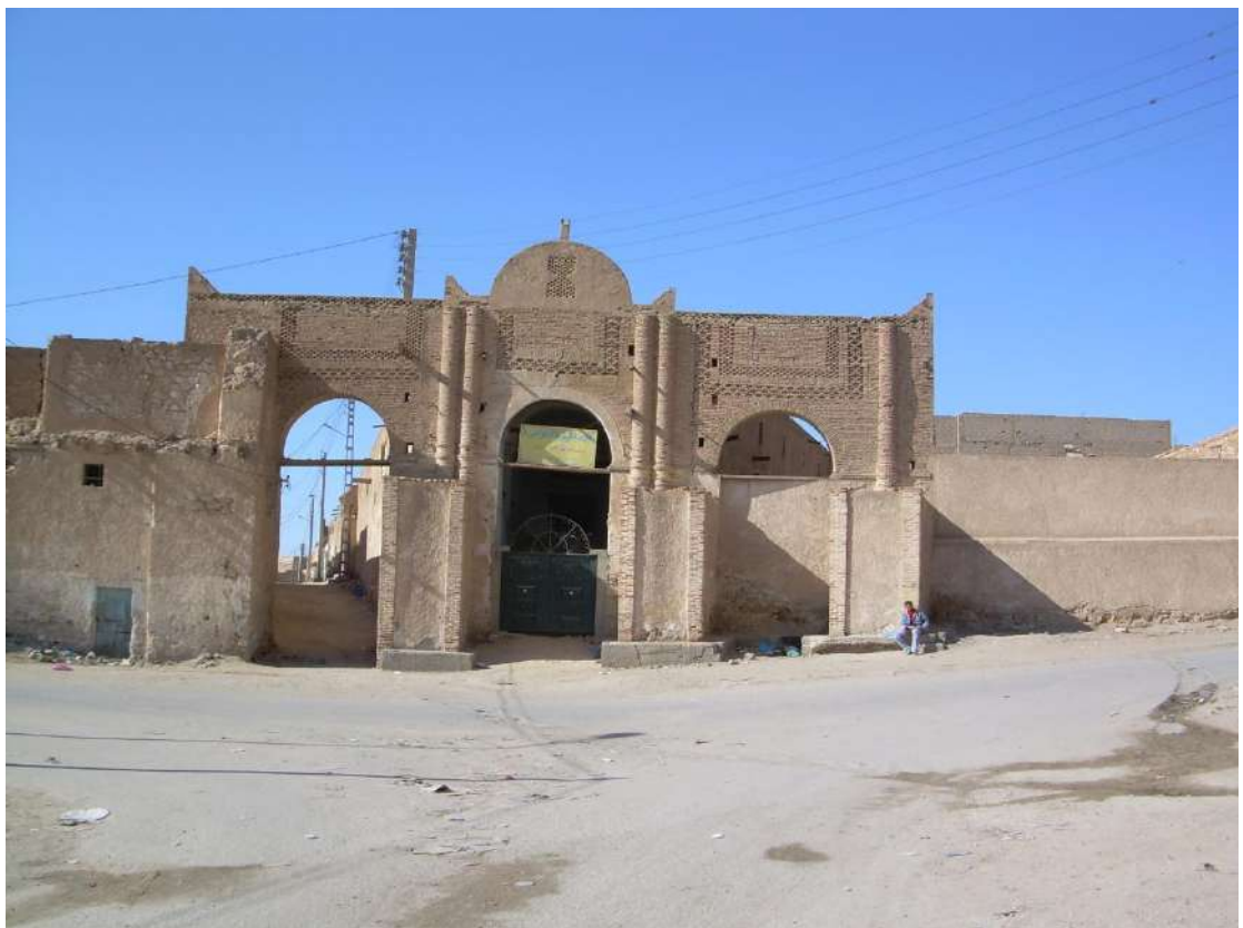
La zaouia Sidi Hachemi, (photo SS, 2010)
